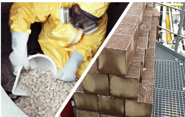
Replacement of ceramic „saddles“ (left) and replacement of ceramic blocks on an RCO incinerator in a cement production (right).
