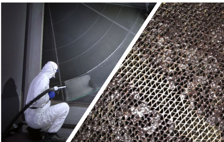
Cleaning of thermal wheel (dia. 5 meters) with dry ice (left); cleaned and uncleaned parts of the honeycomb of a thermal exchanger (right)
